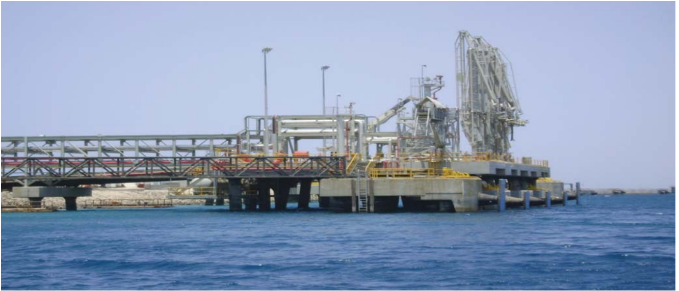
Loading Arm of LNG Terminal at one of the Middle East Country
