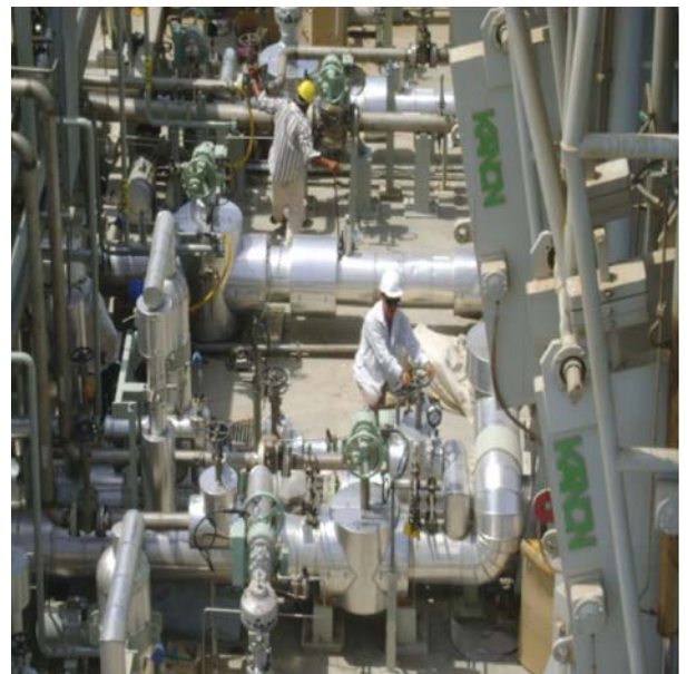
Actual Installation with Heavy Insulation
